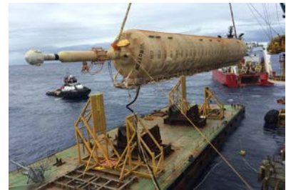
Buoyancy tank being lifted
