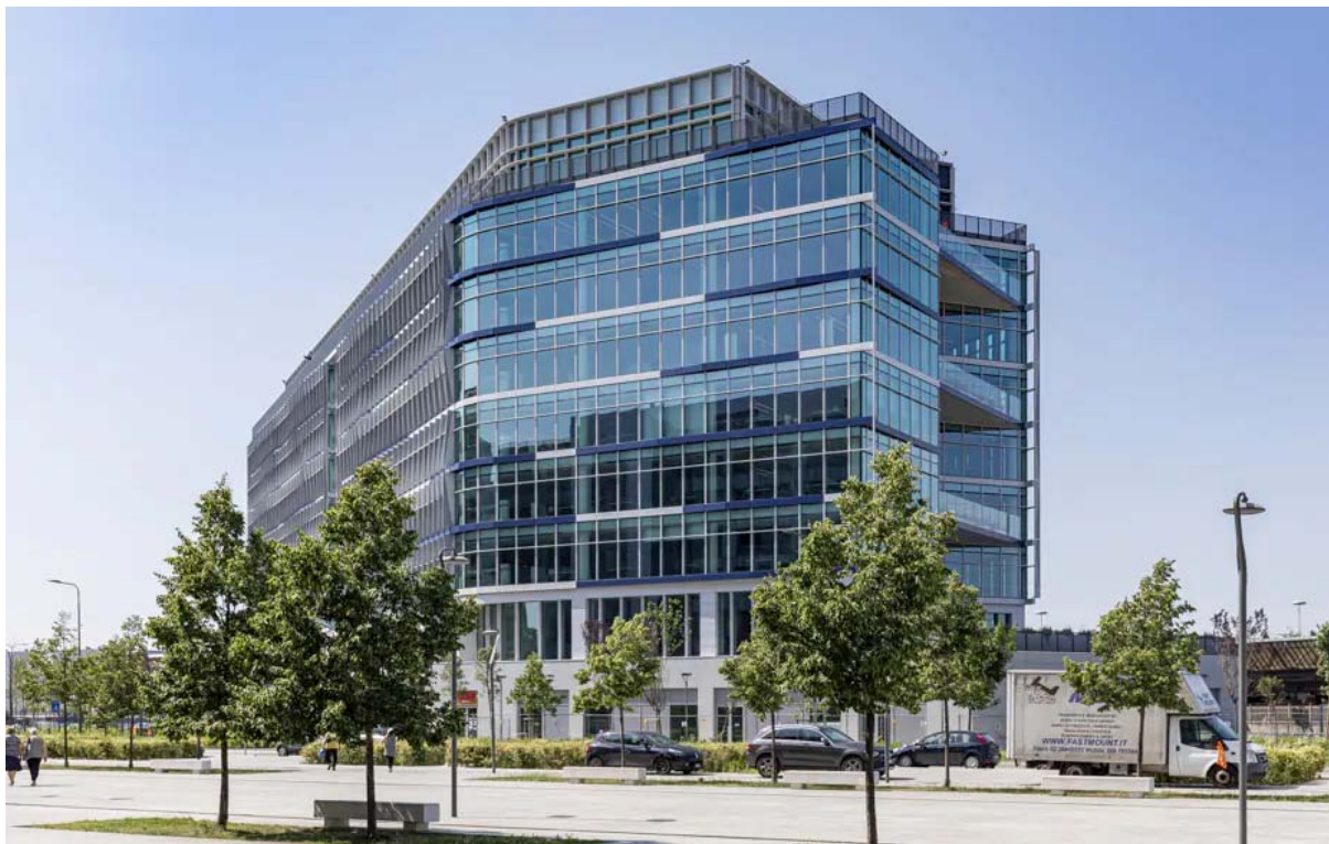
SAIPEM HEAD OFFICE, Spark 1
