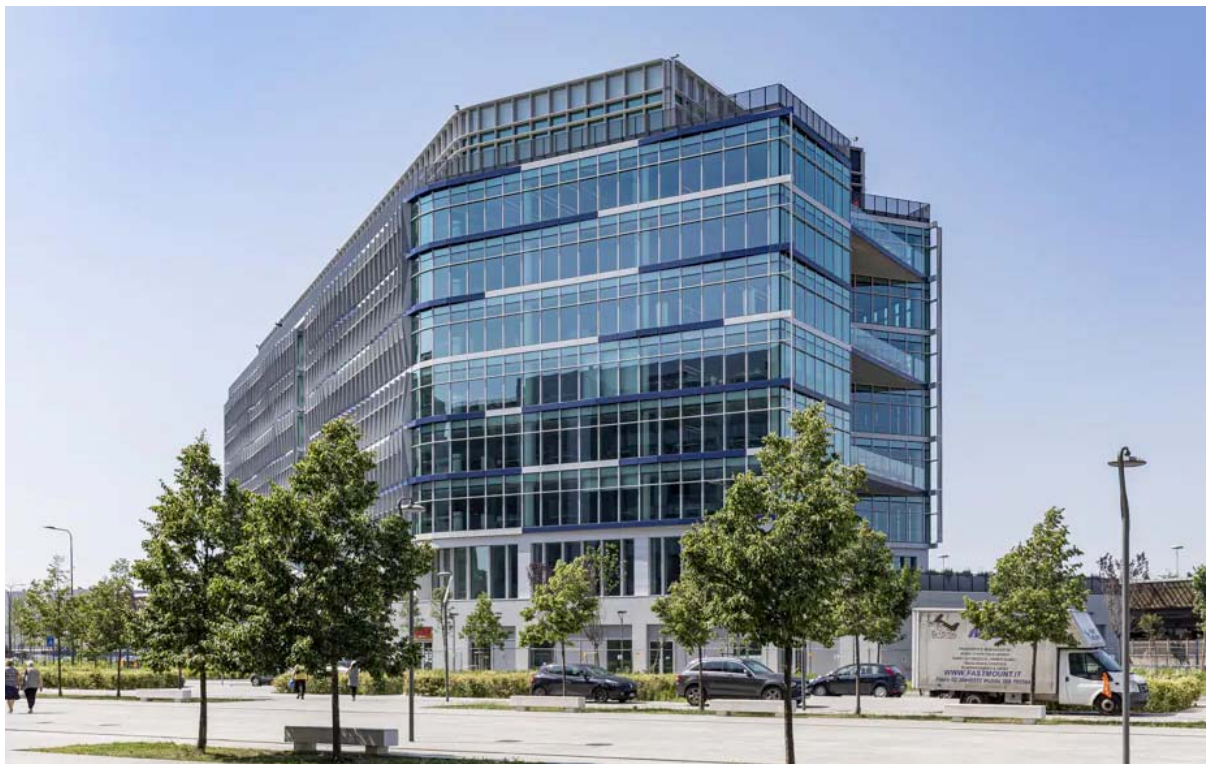
SAIPEM HEAD OFFICE, Spark 1
