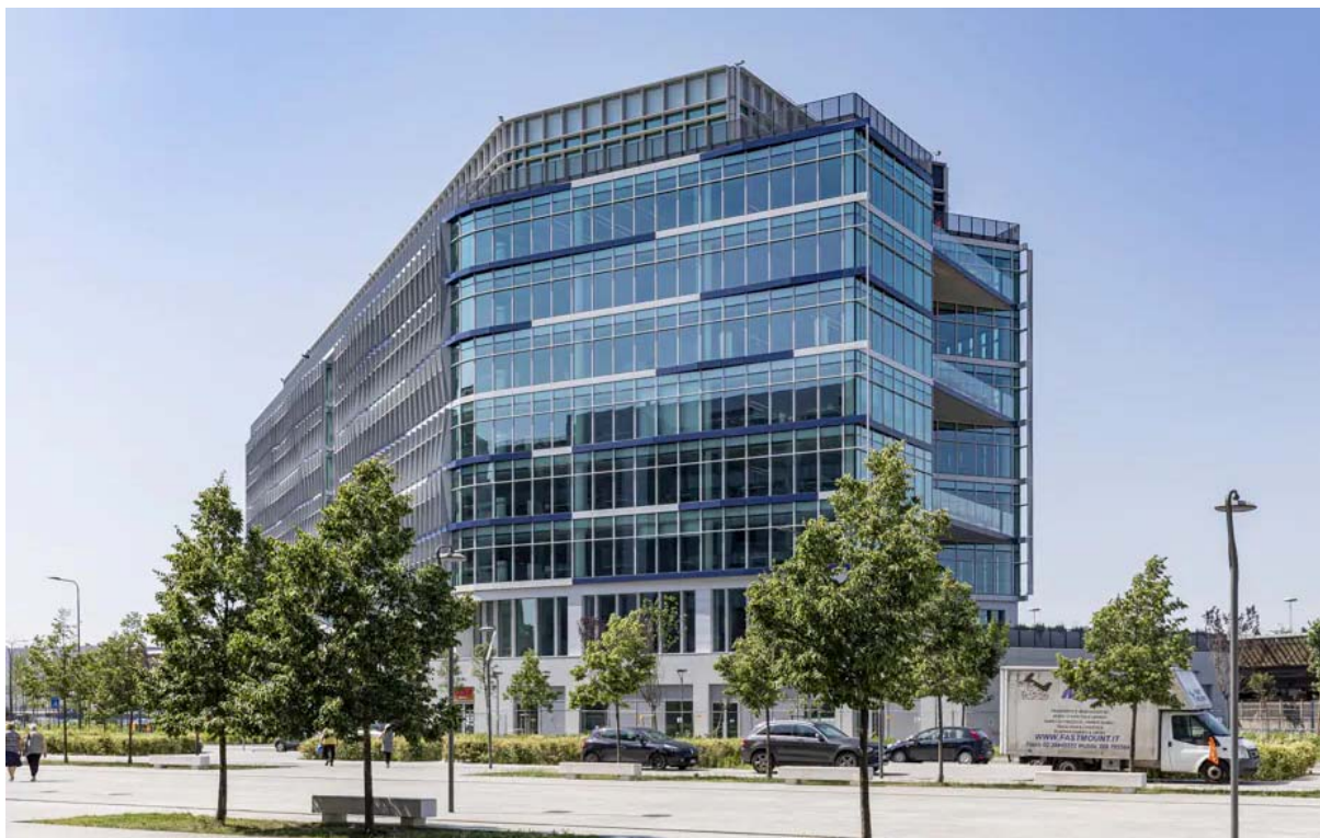
SAIPEM HEAD OFFICE, Spark 1
