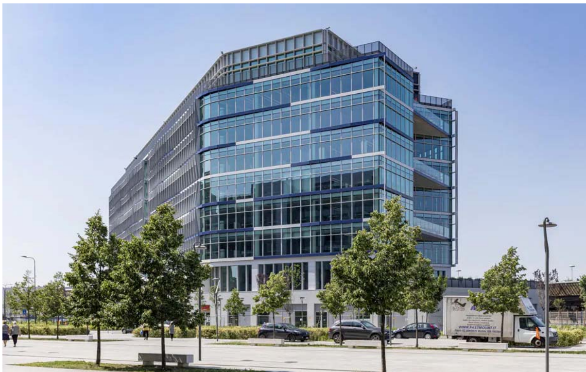
SAIPEM HEAD OFFICE, Spark 1
