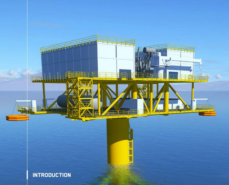
The floating offshore wind farms are becoming the more interesting and economic solution for sites with 60 m of water depth. While several designs for floating foundations for Wind Turbine Generators have been developed and patented, floating substations are representing the next step to have a complete solution for a floating wind farm applicable to a large panel of site conditions and characteristics.
