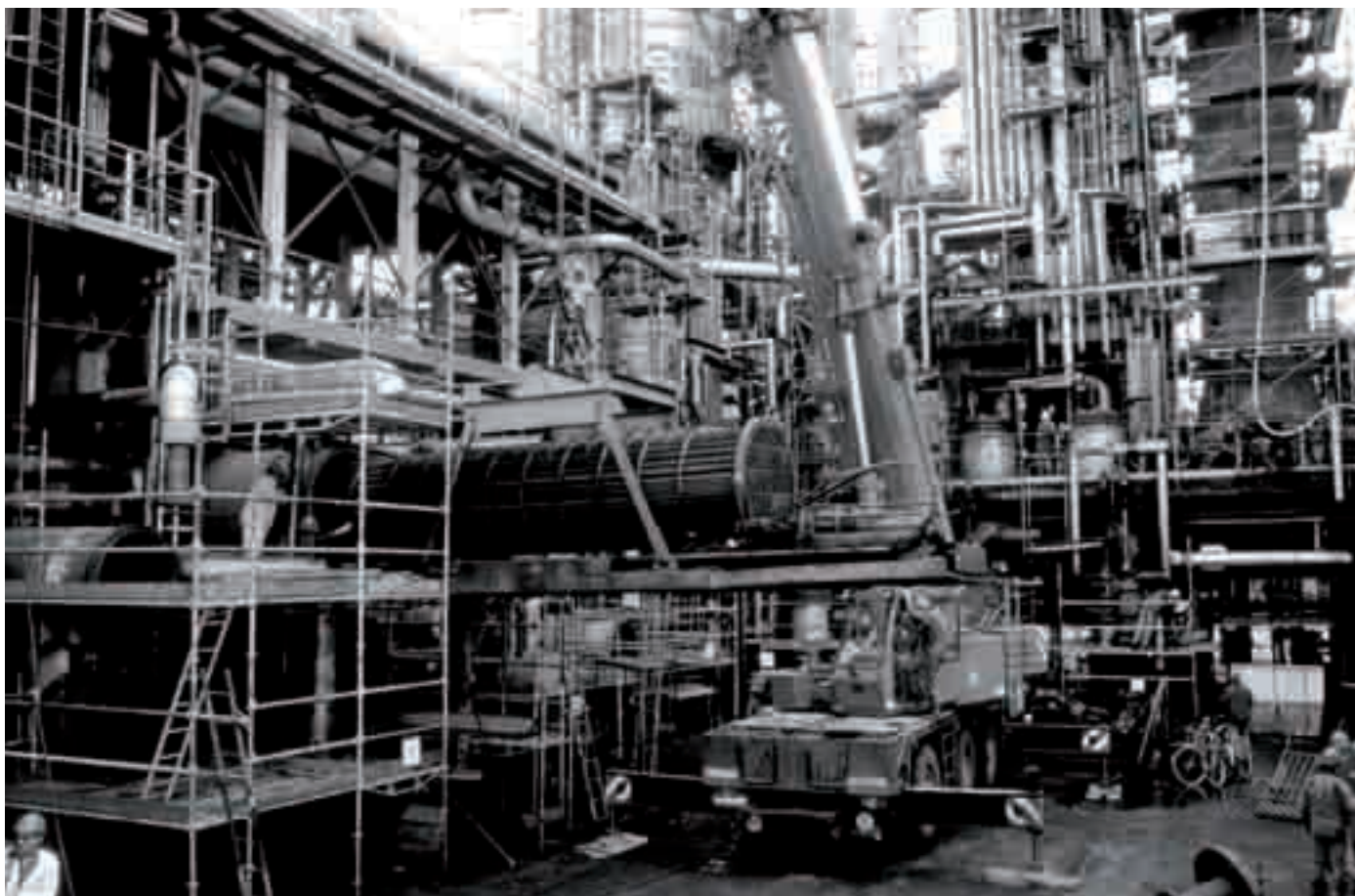
Refinery shutdown/turnaround in the 80's
