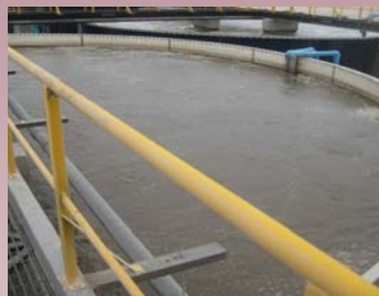
Phase 3 Aeration Tank
