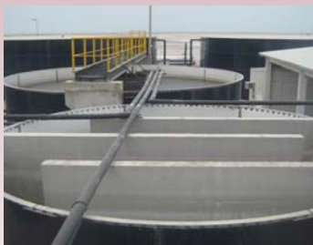
Phase 5 Chlorination Tank
