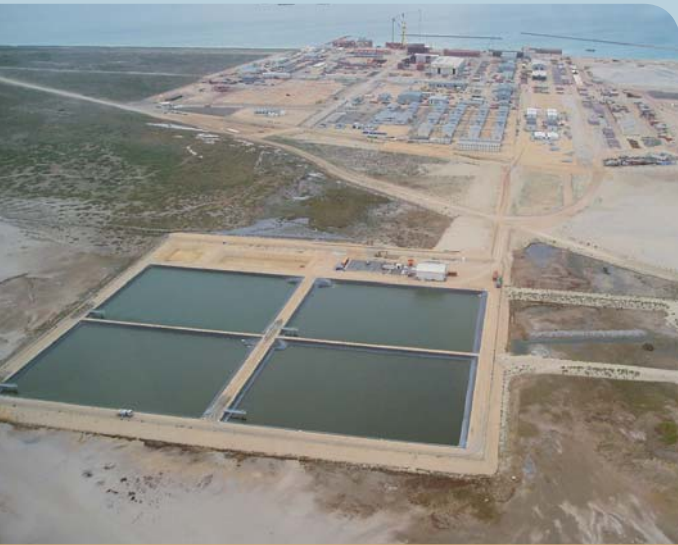
Ersai waste water treatment plant
