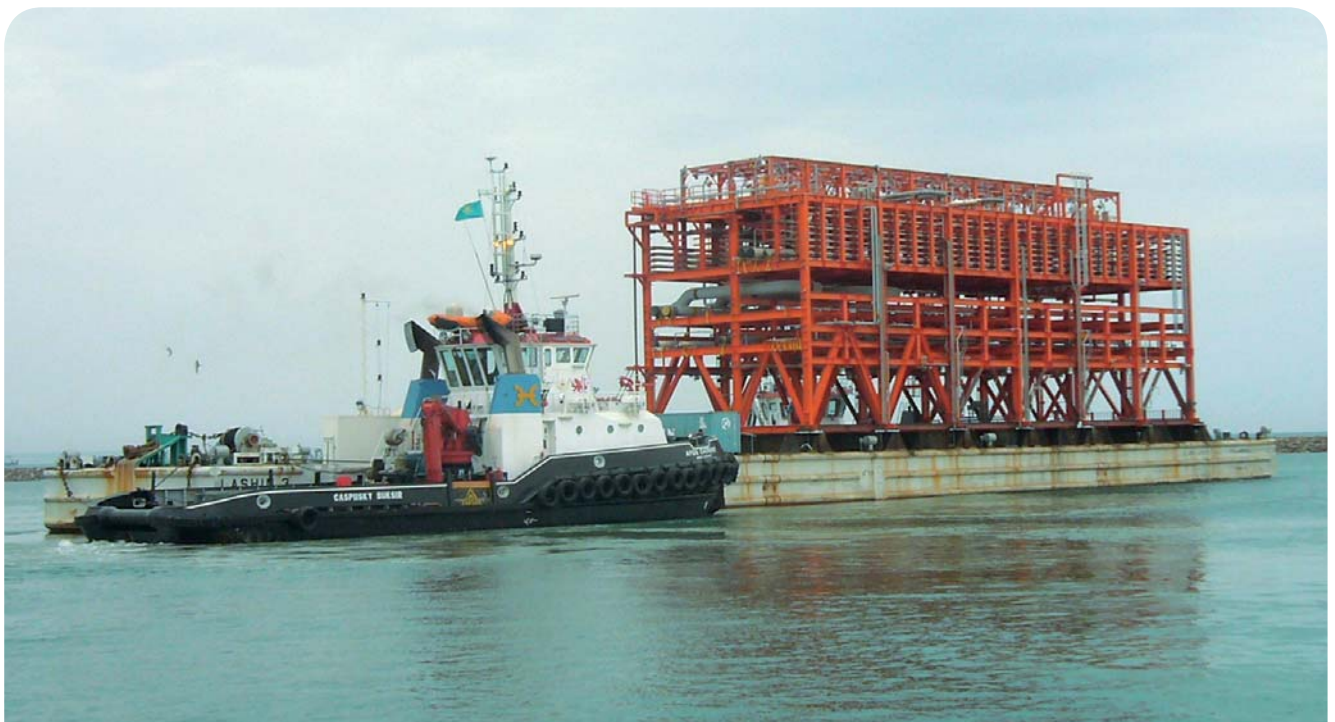
Sail away of Pipe Rack 5.1
