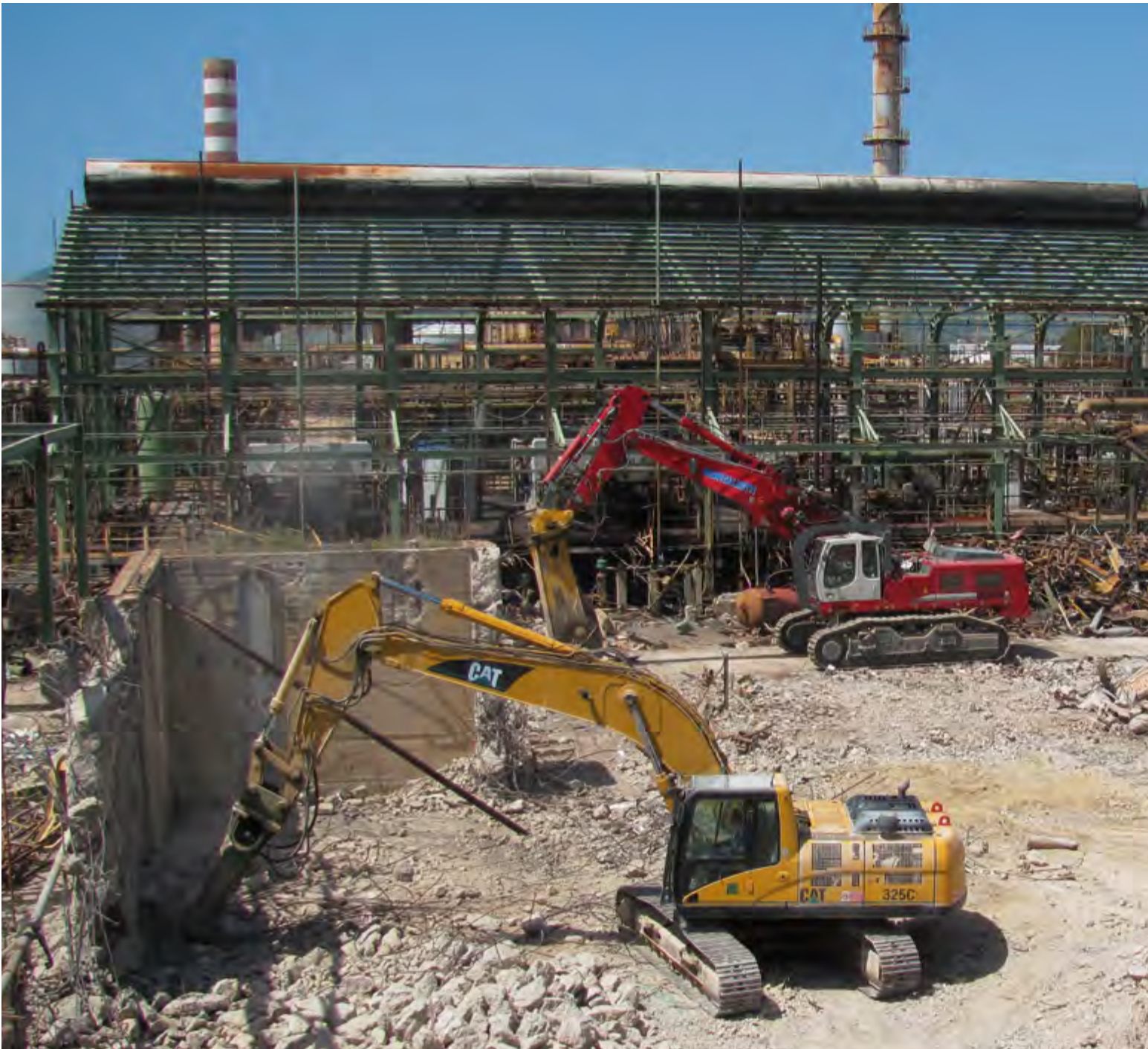
Assemini Plant Dismantling
