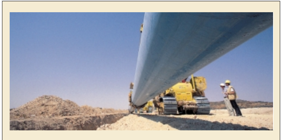
Saudi Arabia, the laying of a pipeline.
