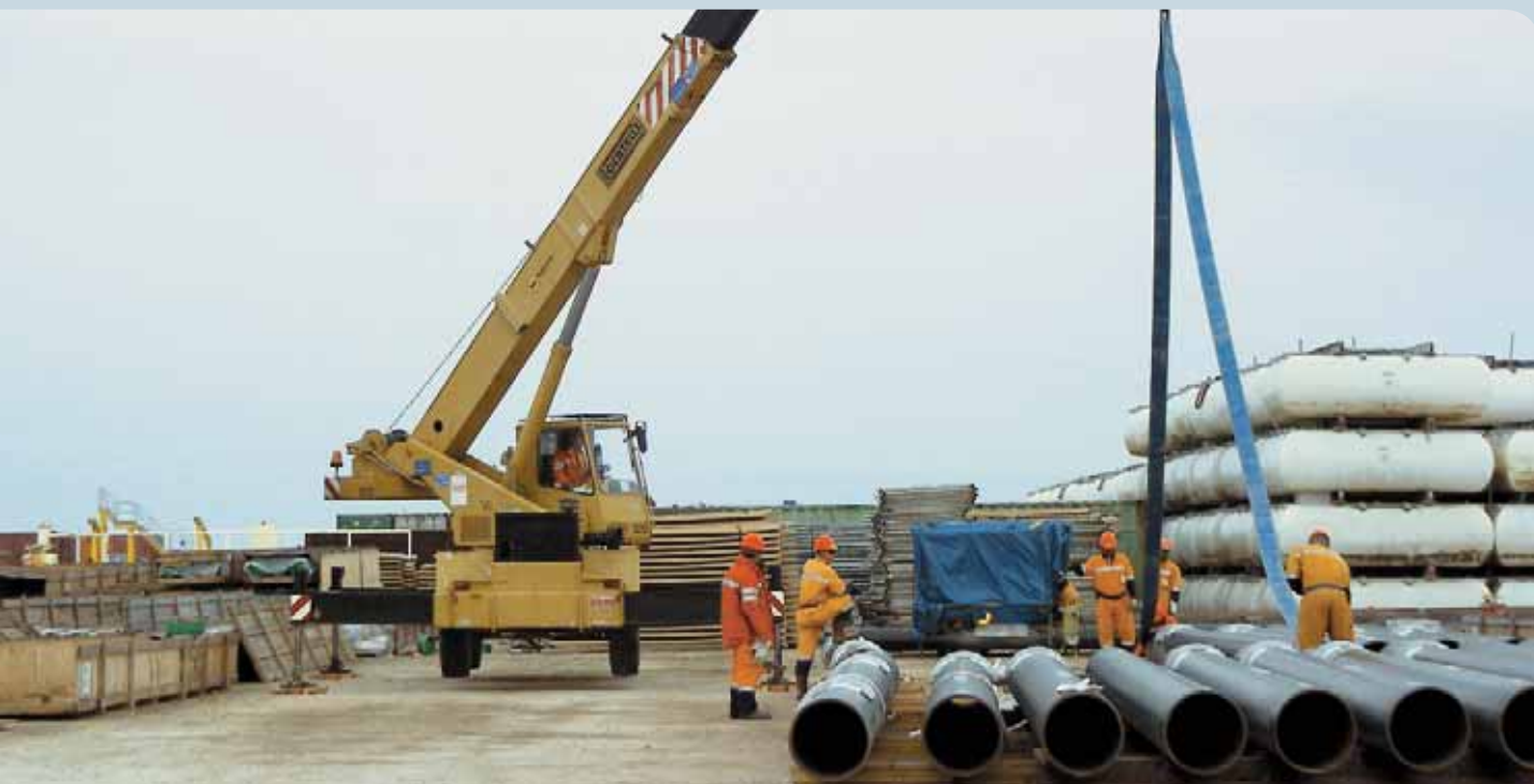
Bibigul Kashabayeva - Preparation of the pipes for transportation offshore
