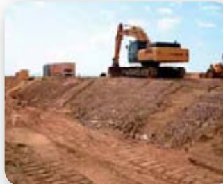
Re-instatement of near shore
