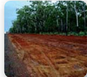
Re-instatement of pipeline corridor
