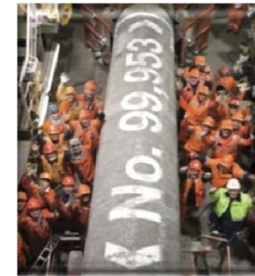
Castoro Sei: launch of Nord Stream last pipe
