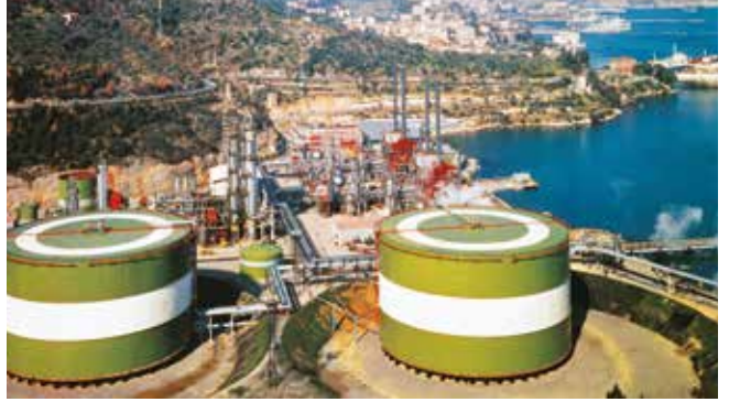
Panigaglia LNG regasification plant in Italy for SNAM S.p.A. (1971)
